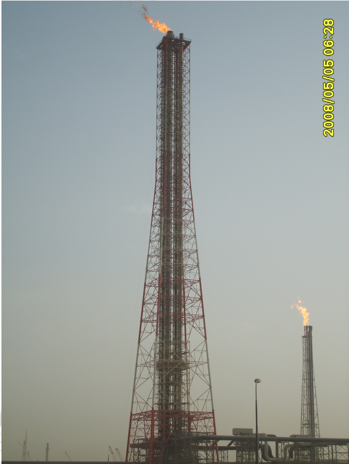
200m Height Demountable Flare - Qatar
