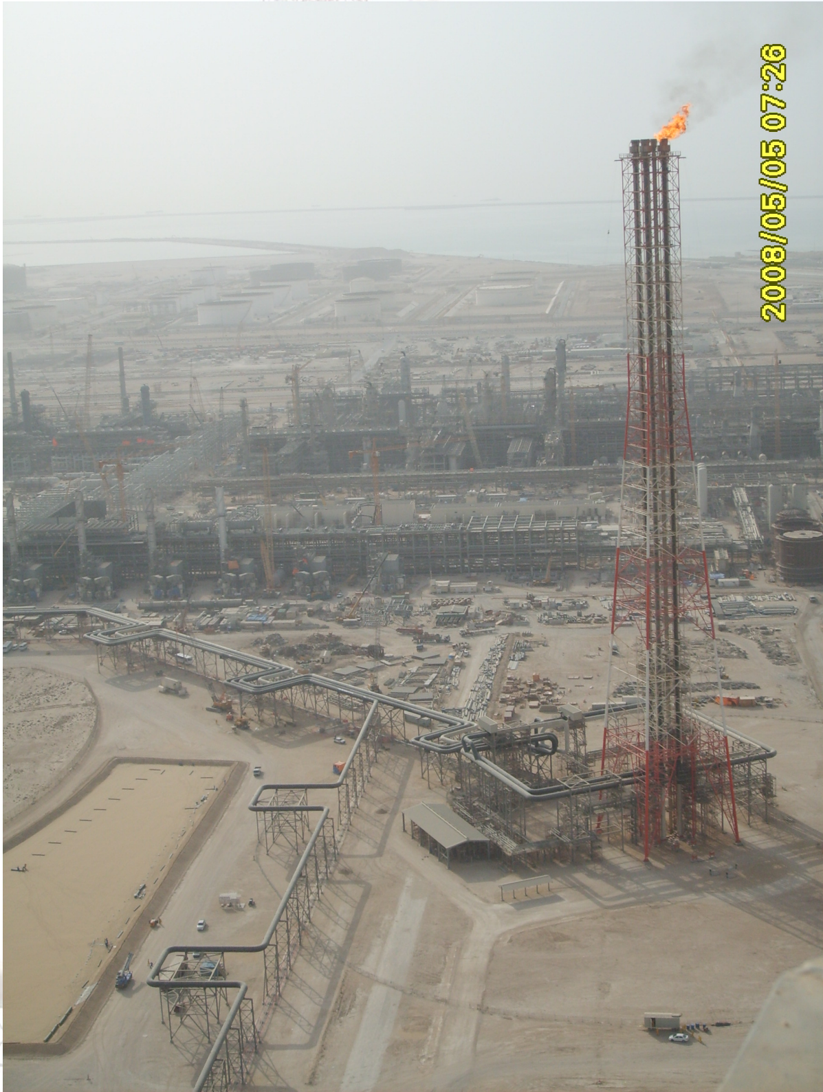
200m Height Demountable Flare - Qatar
