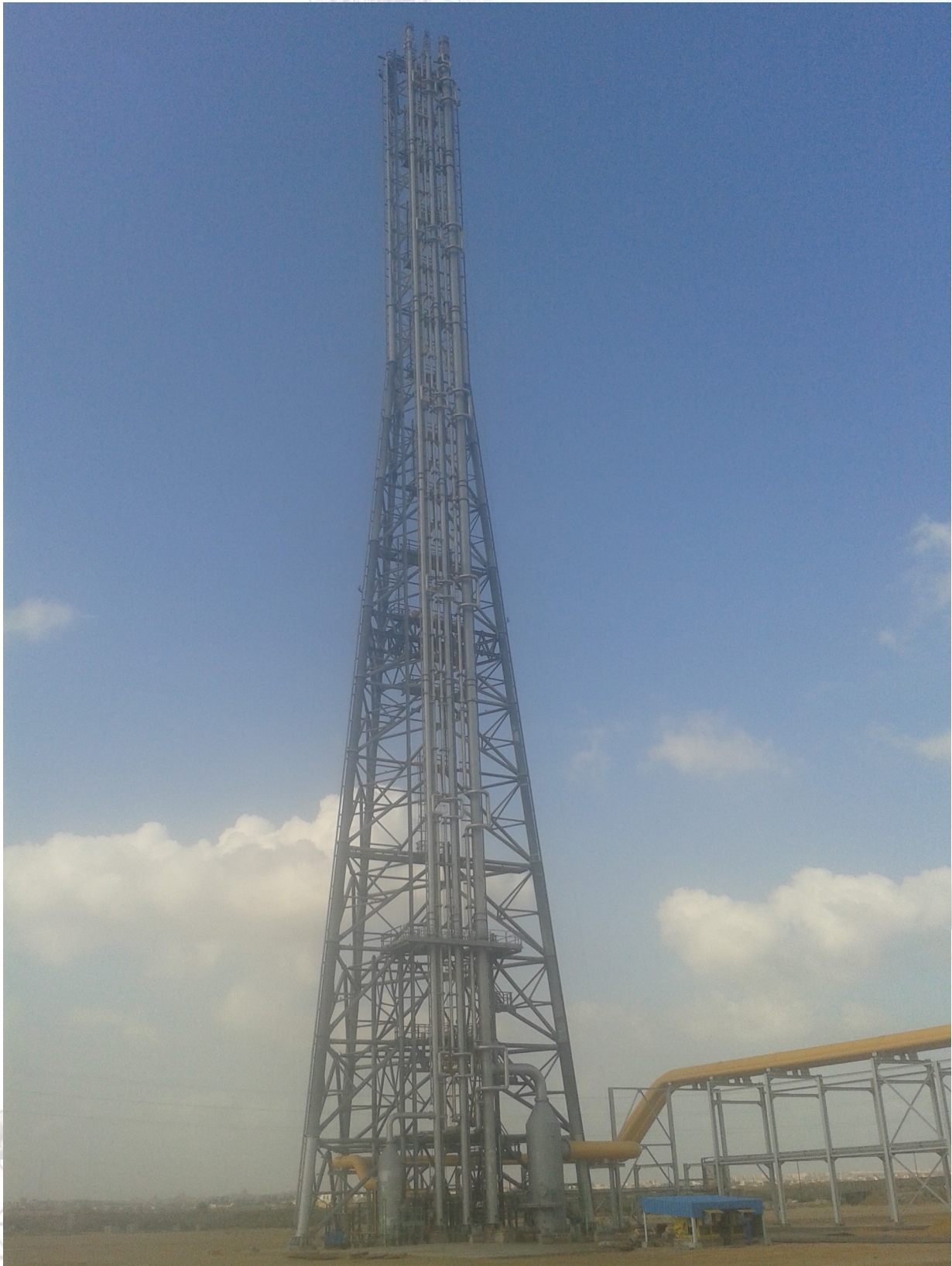
126m Height Demountable Flare – Egypt
