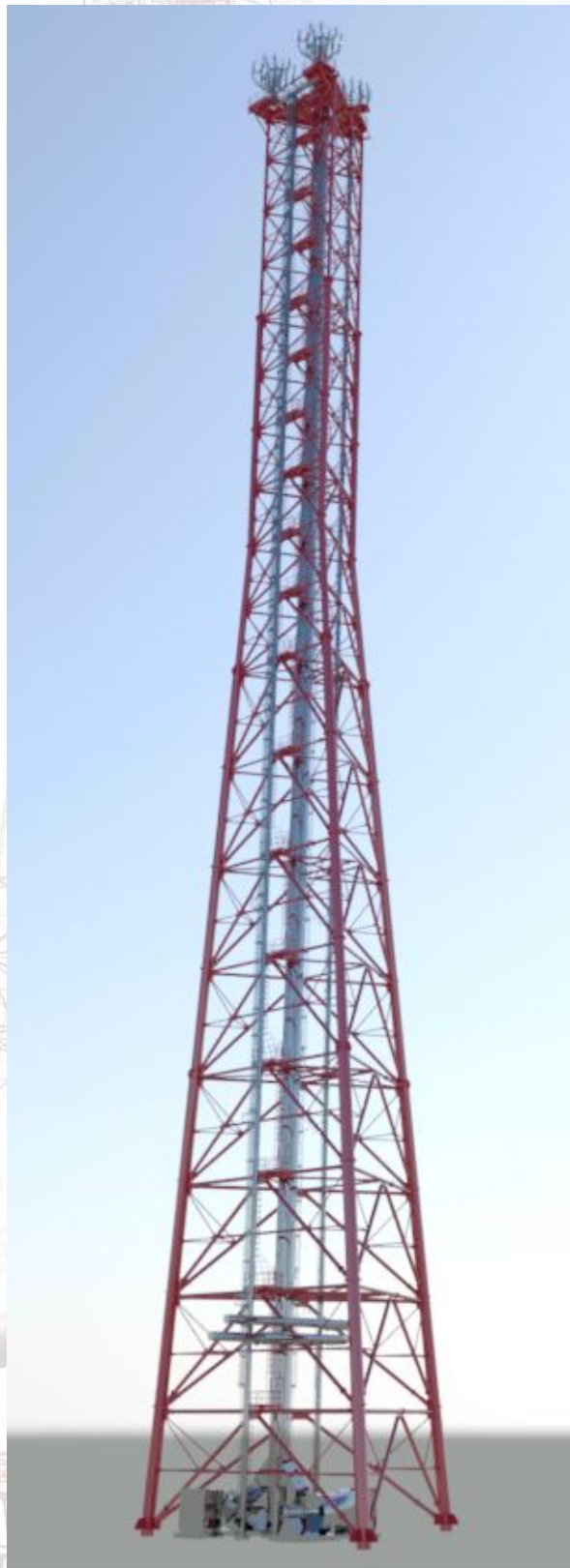
136m Height Fixed Flare – Temparossa Italy
